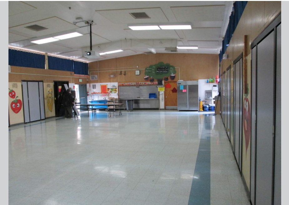
Multi-purpose room interior finish upgrades
