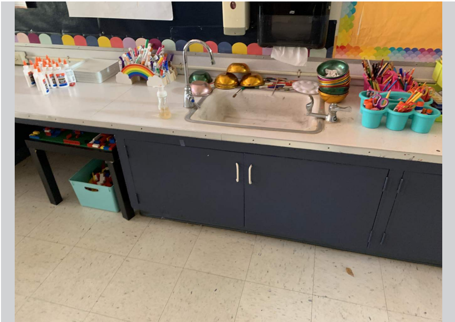
ADA compliant accessibility improvements to sink areas
