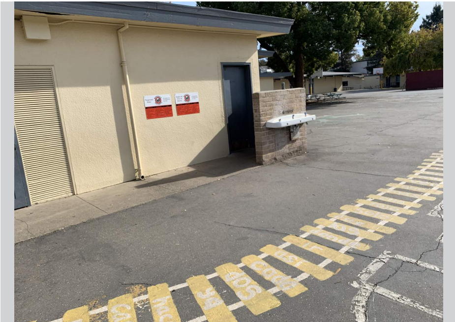
Water fountain upgrades
