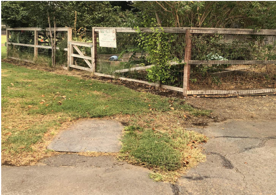
ADA path of travel improvements to pavement and landscape
