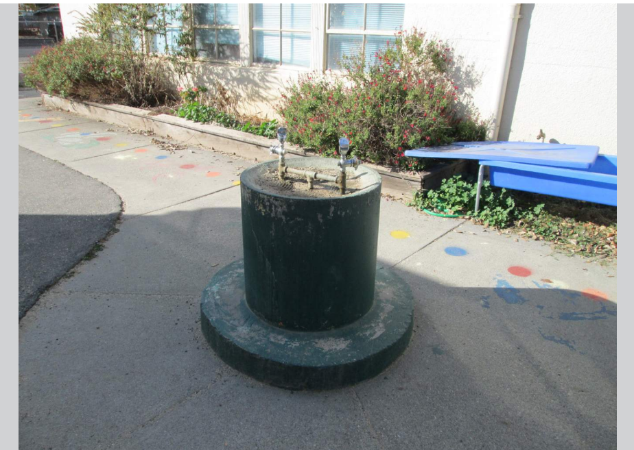
Exterior water fountain replacement
