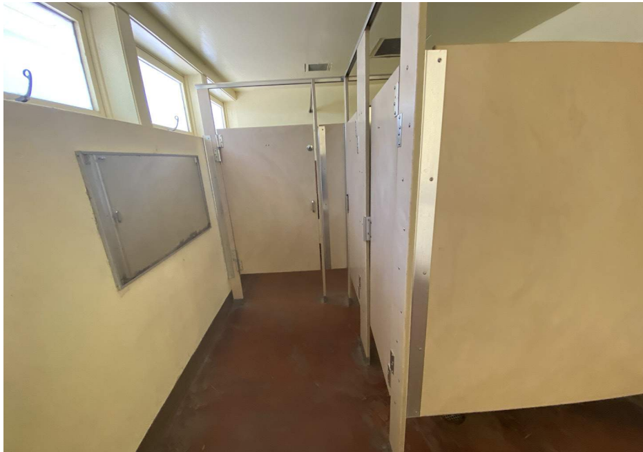
Core restroom ADA compliance upgrades
