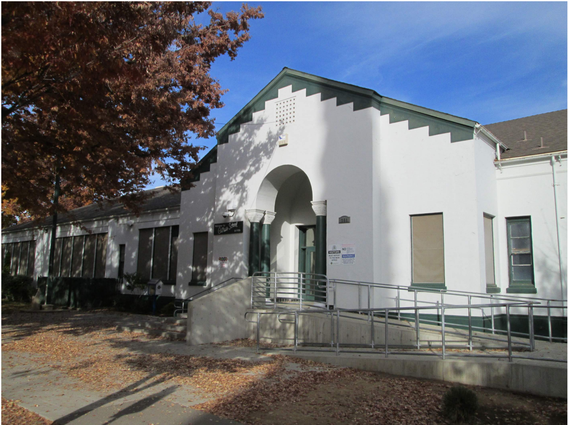
Entry and multipurpose at Chapman Elementary School.
