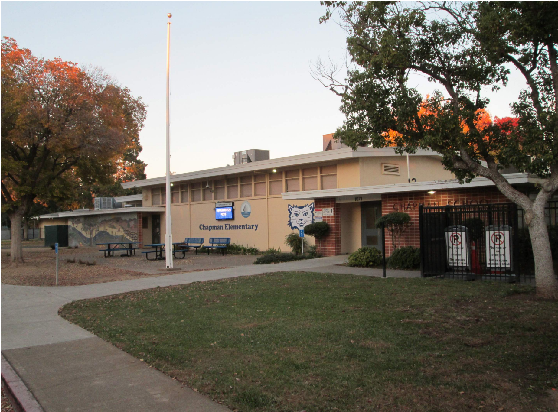
Entry and multipurpose at Chapman Elementary School.
