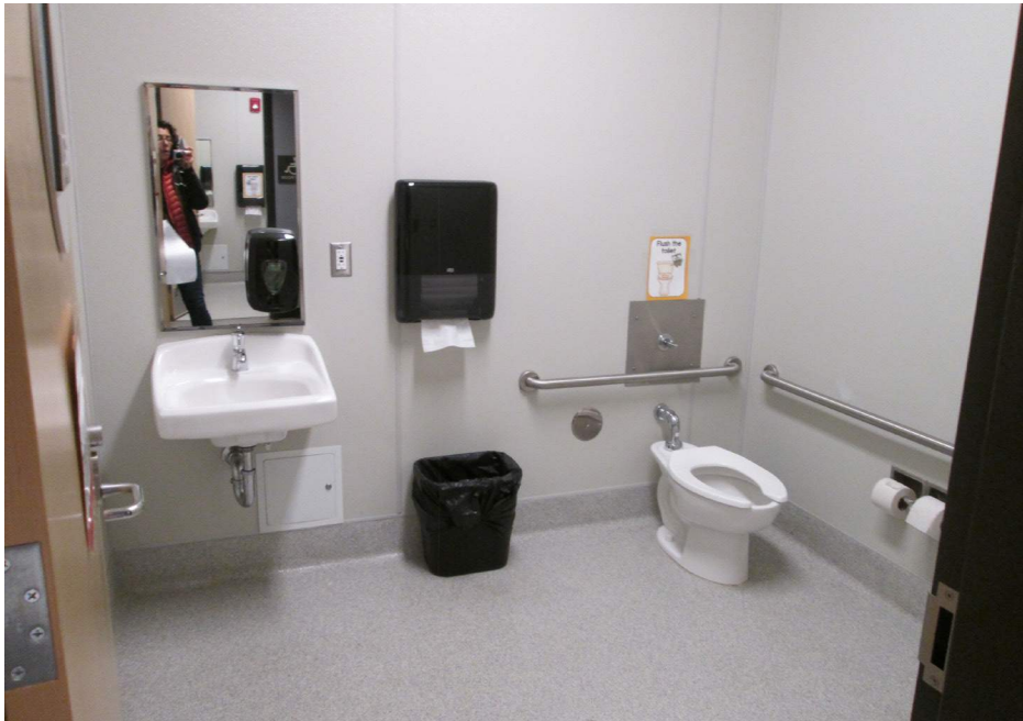
Restroom finishes and fixtures
