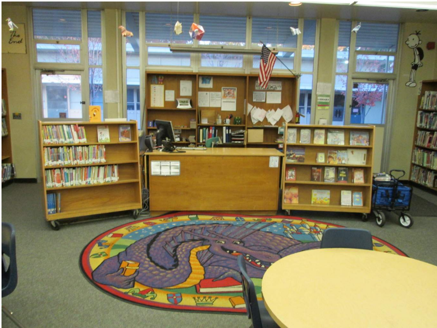
Aging casework and finishes
