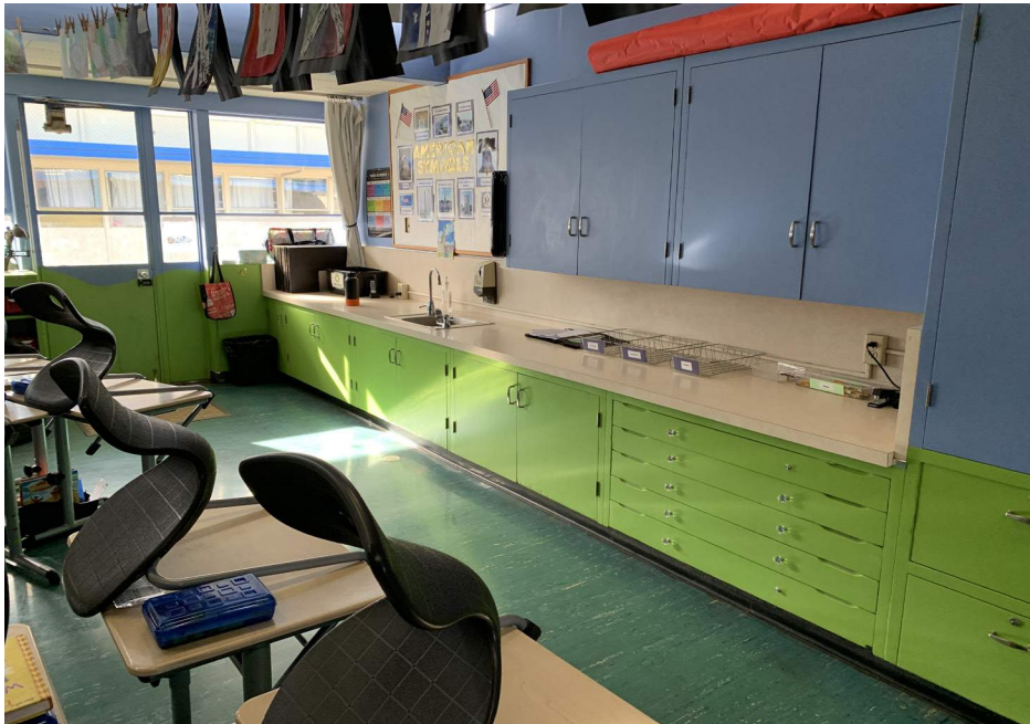
Casework replacement and ADA upgrades
