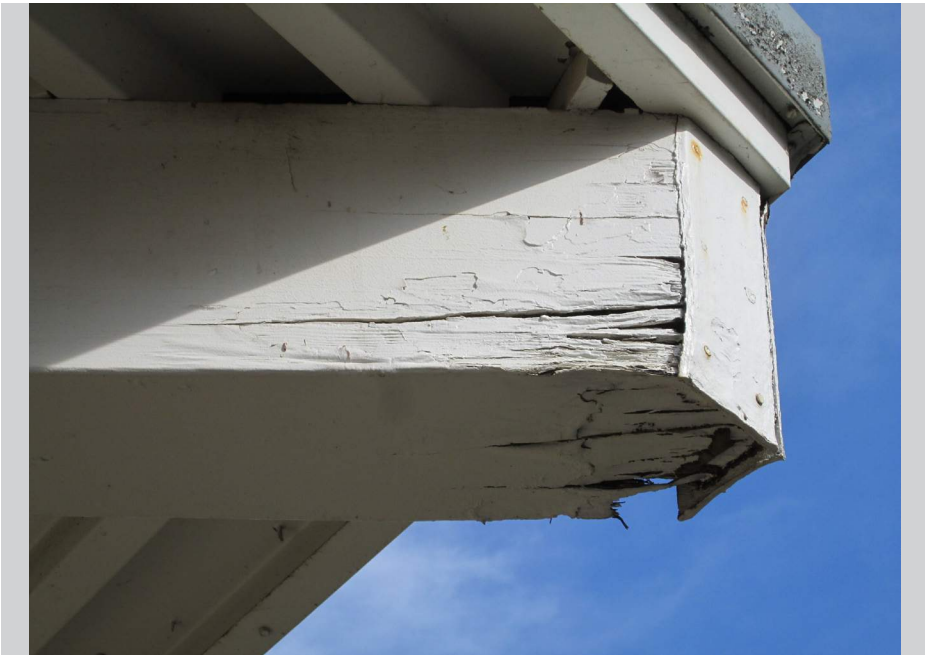
Exterior soffit and fascia replacement
