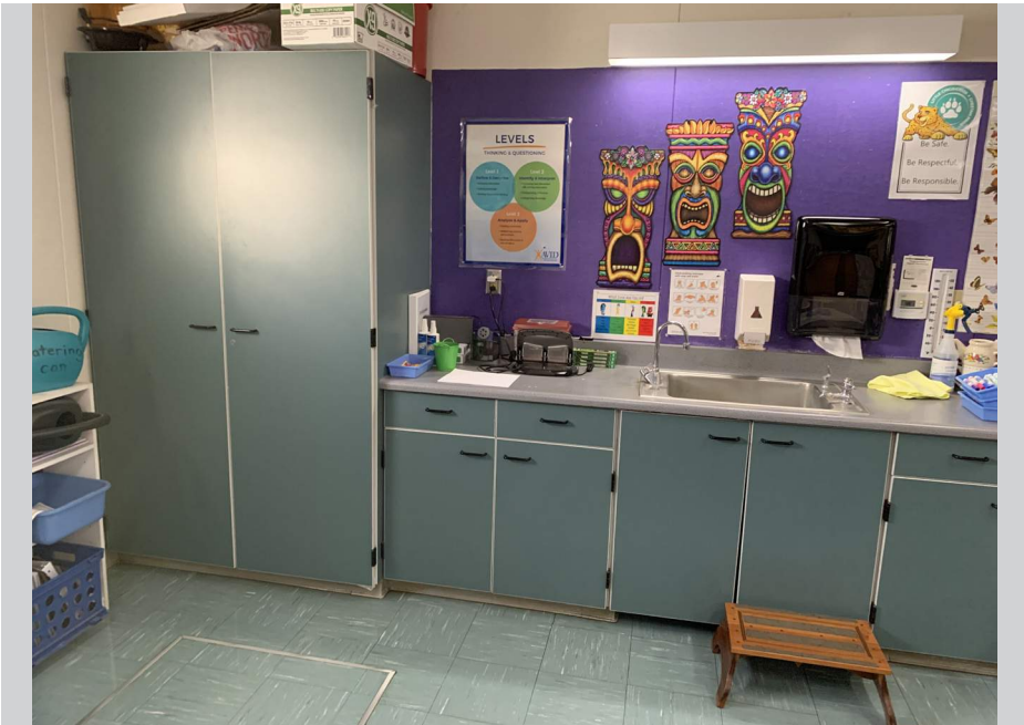
Casework and sink replacements for ADA compliance
