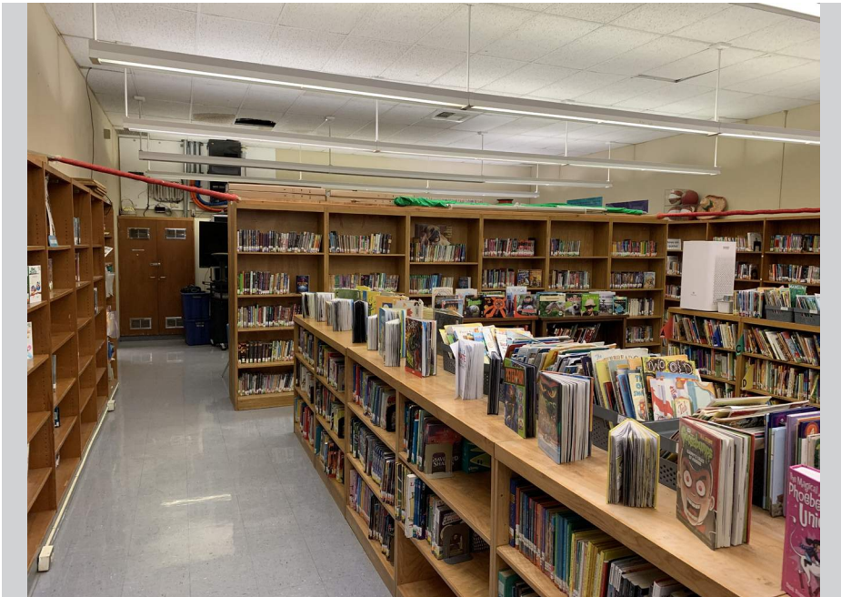
Campus library electrical improvements
