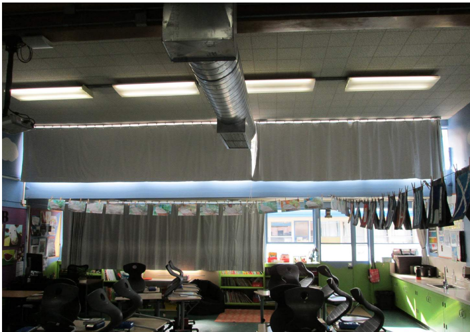
Classroom clerestory and window treatment upgrades
