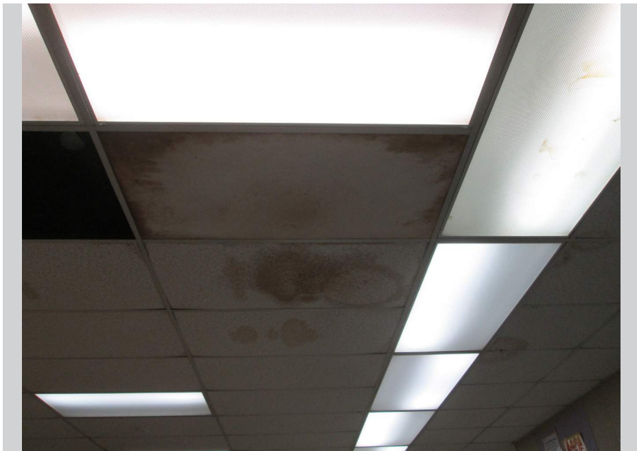
Acoustical Ceiling Tile replacement
