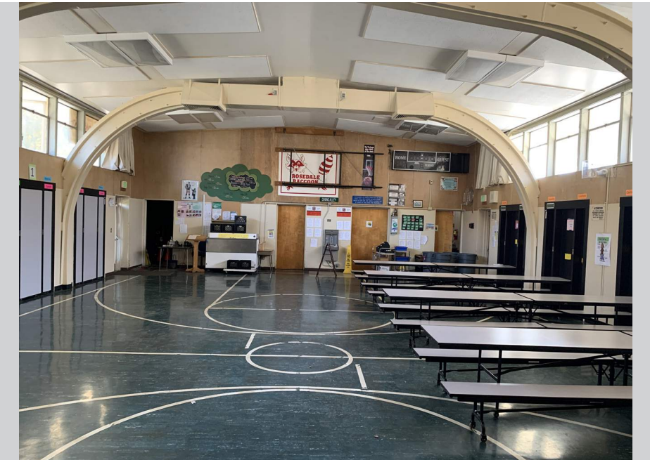
Multi-purpose interior finish renovations and storage improvements
