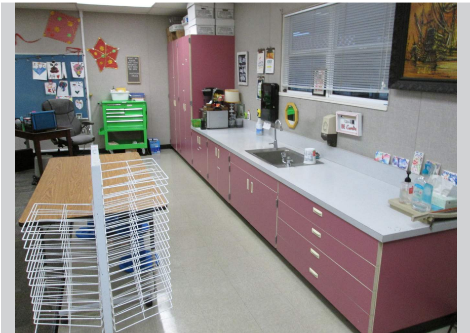
Casework and sink improvements for ADA compliance
