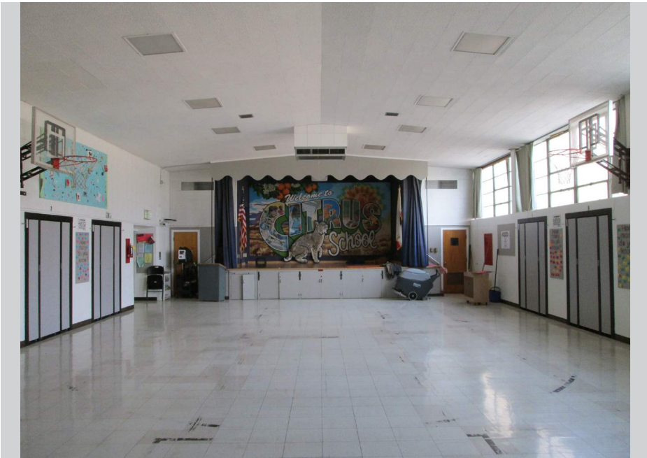
Multi-purpose room renovation and storage improvements
