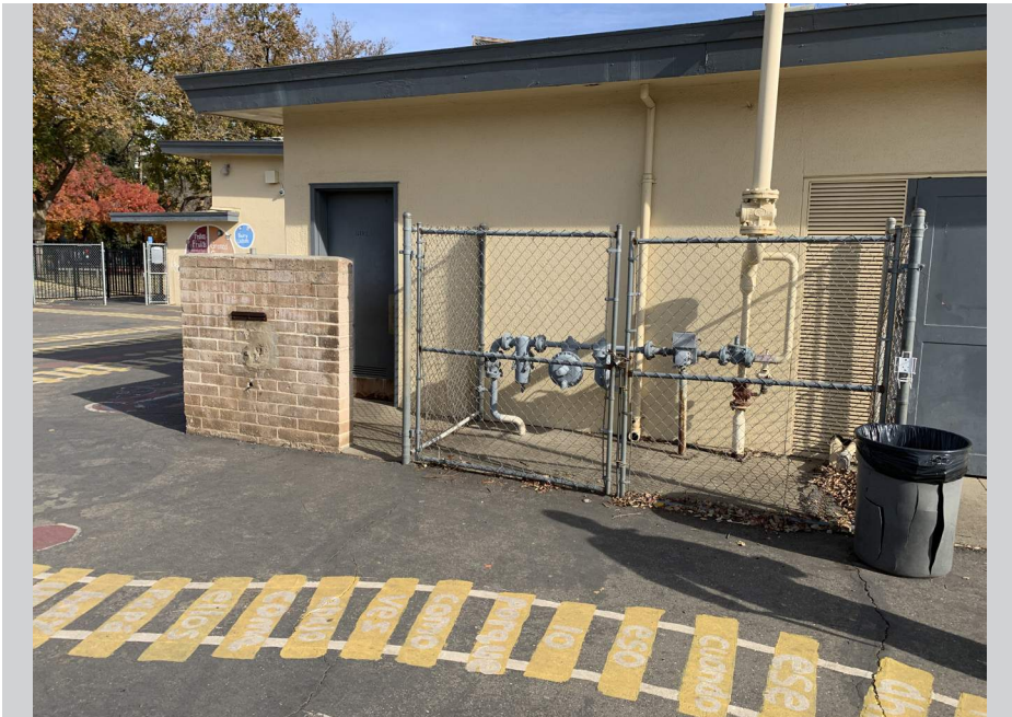
ADA accessibility improvements
