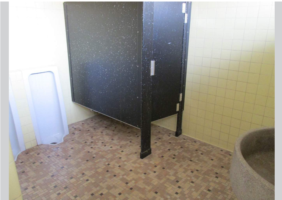
Student restroom ADA upgrades and renovations
