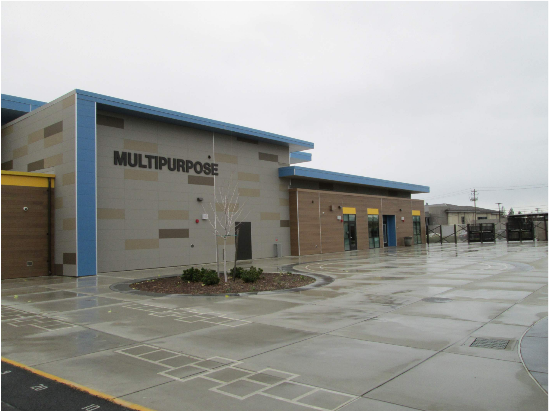
Entry and multipurpose at Marigold Elementary School.
