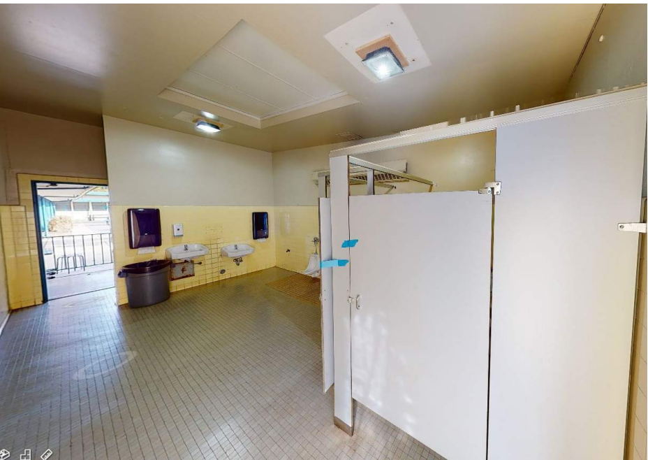
Student restroom interior finish upgrades
