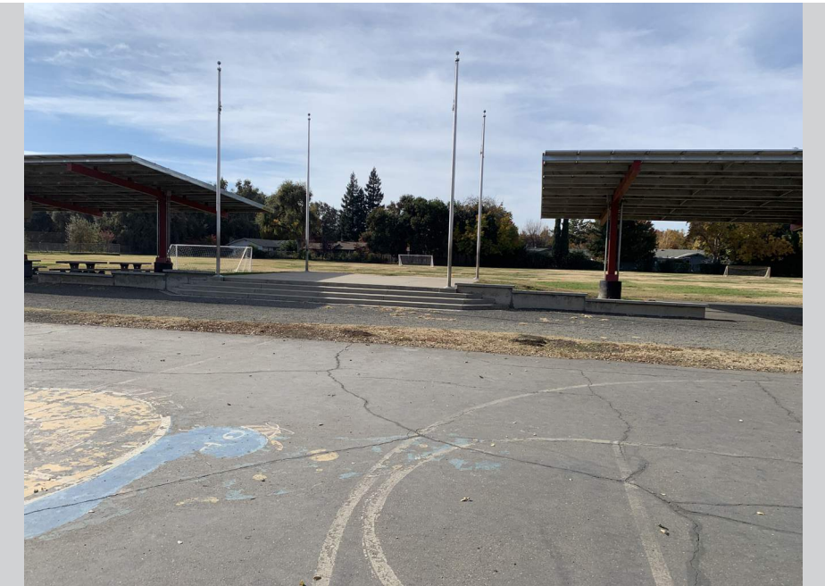
Landscape improvements and hardcourt repavement
